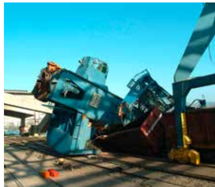
A harbour crane broke off after the tower rusted through
